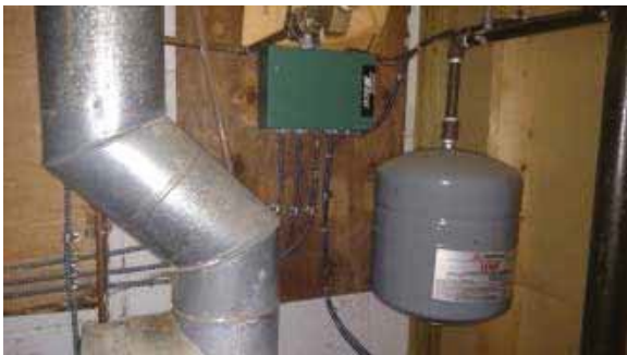
MI.3 - Flue From Boiler
