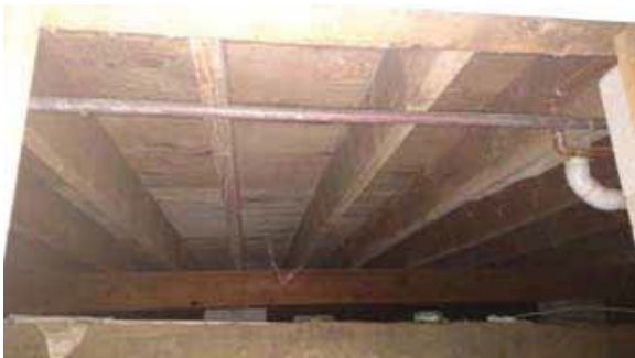
MI.5 - Uninsulated Piping in Crawl Space
