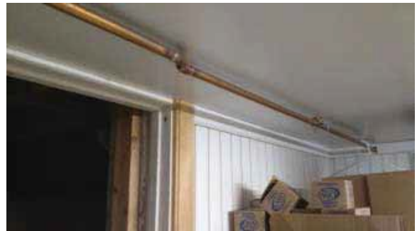
MI.6 - Uninsulated Supply Piping
