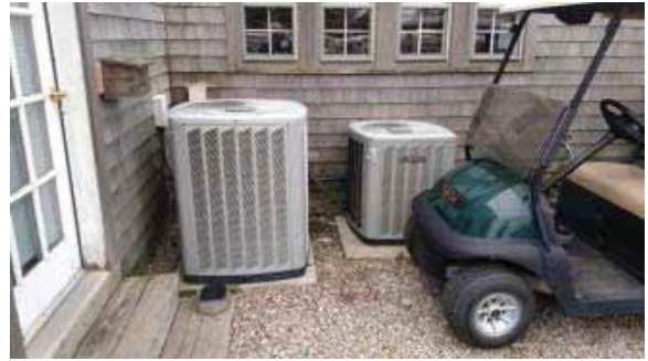
M2.2 - Air Cooled Condensing Units
