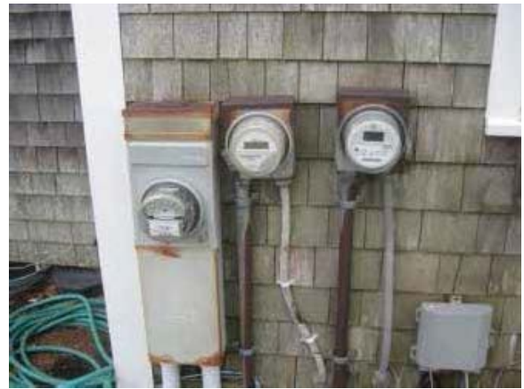
EI.8 – Poorly Maintained Utility Meters
