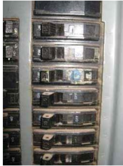
El.4 - Corroded Circuit Breakers
