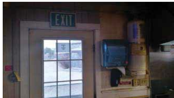
FPI.4 - Hood Extinguisher Button (Left of Door)
