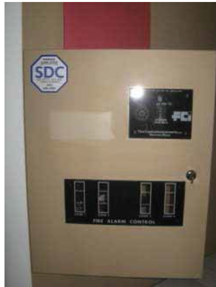
E2.4 - Fire Alarm Control Panel
