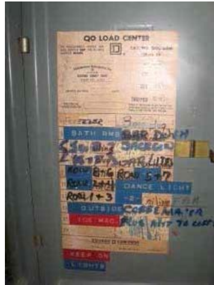
EI.6 – Poorly Maintained Panel Schedule
