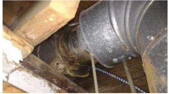
MI.8 – Corroded Boiler Flue
