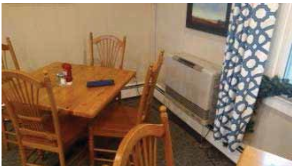
MI.13 – Direct Fired Propane Heater
