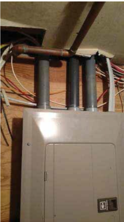
MI.9 – Water Piping Above Electrical Panel
