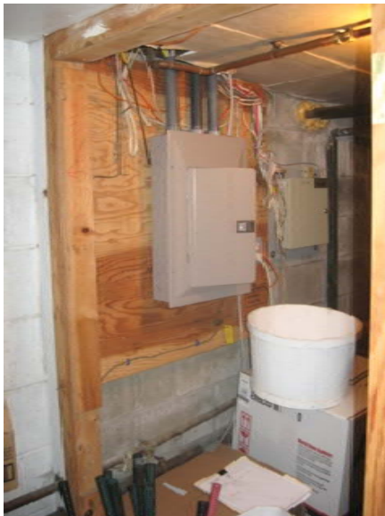
El.3 - Panel with water pipe routed above
