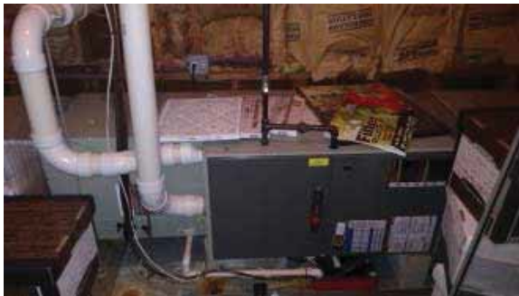
M2.3 - Typical Air Handling Unit and Cooling Coil
