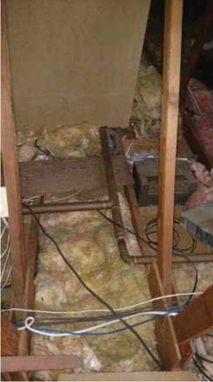
PI.14 – Plumbing Vent piping in Attic
