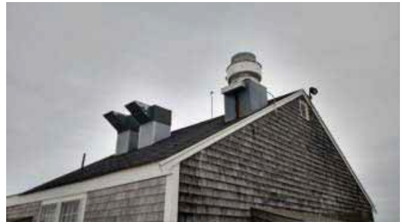
MI.2 -Fresh Air Intake and Exhaust for Hood
