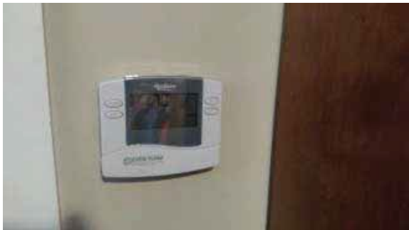
M2.5 - Typical Wall Thermostat
