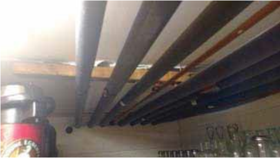
MI.7 – Poorly Hung Piping in Basement
