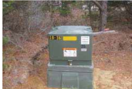
E4.6 - Transformer for Indoor Golf Cart Storage
