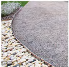
STONE DUST SURFACING WITH METAL EDGE
